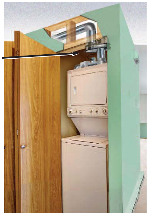
Typical Closet Installation
